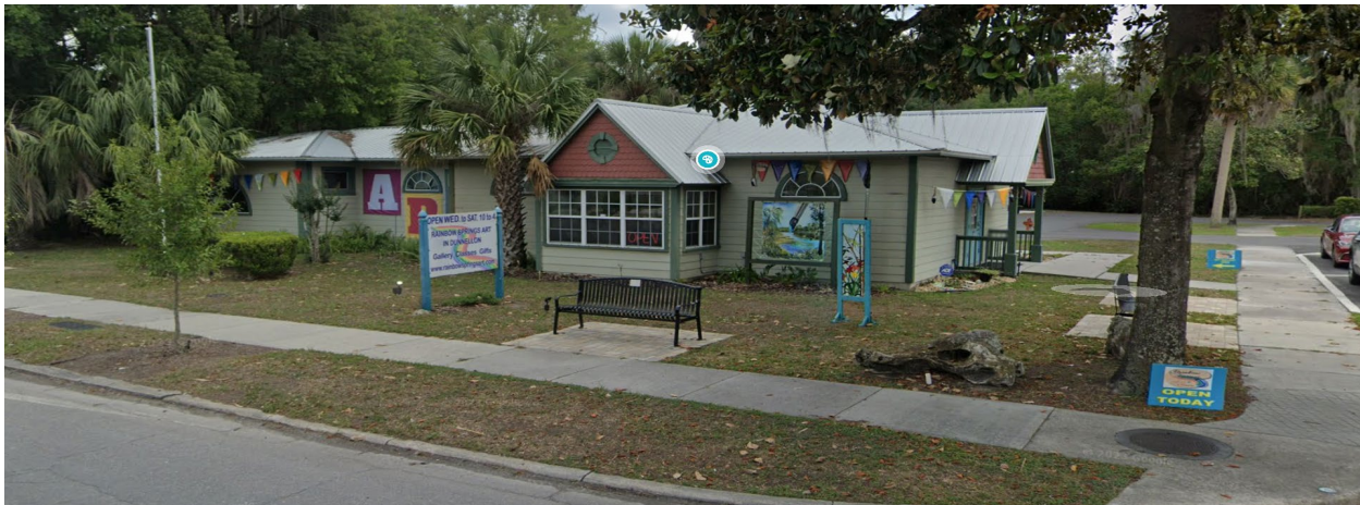
20804 W Pennsylvania Avenue – View from Pennsylvania Avenue
